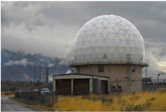
Figure 8.13: The AN/FPS-117 engineering facility at Hill Air Force Base, Utah, one of the DoD 5G testing sites 123
